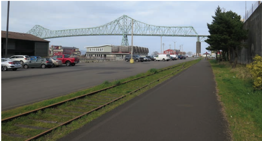
Figure 14: Riverwalk Trail (foreground) and large parking lot
