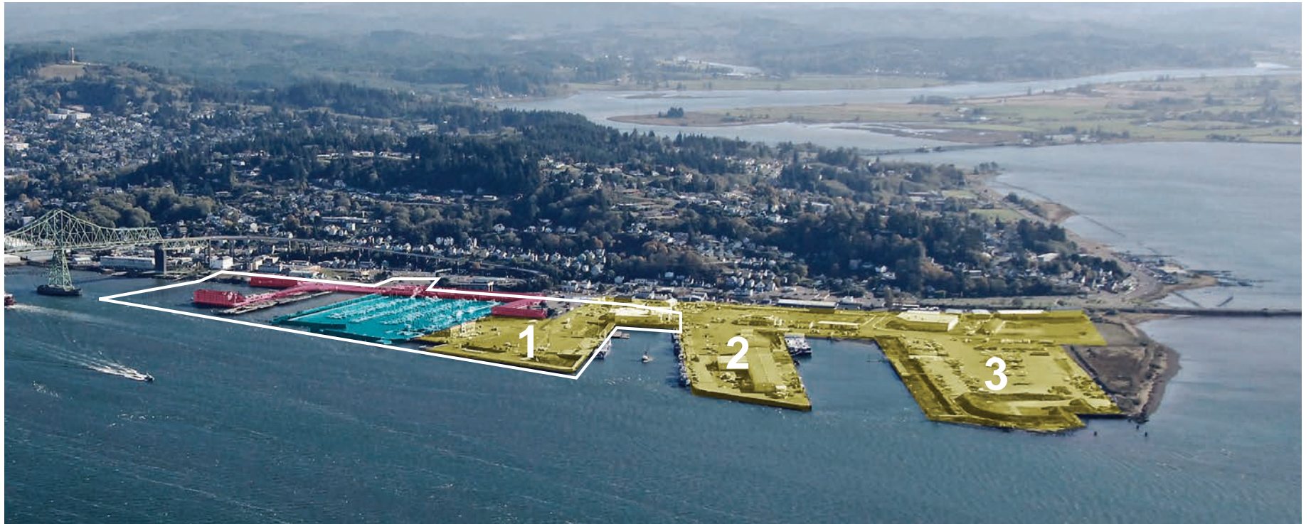
Figure 7: Study area in context; Piers 1, 2, and 3
